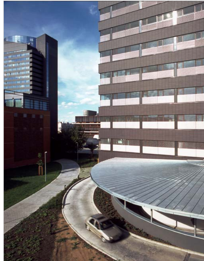
Entrance to underground car park at Budejovicka Alej
